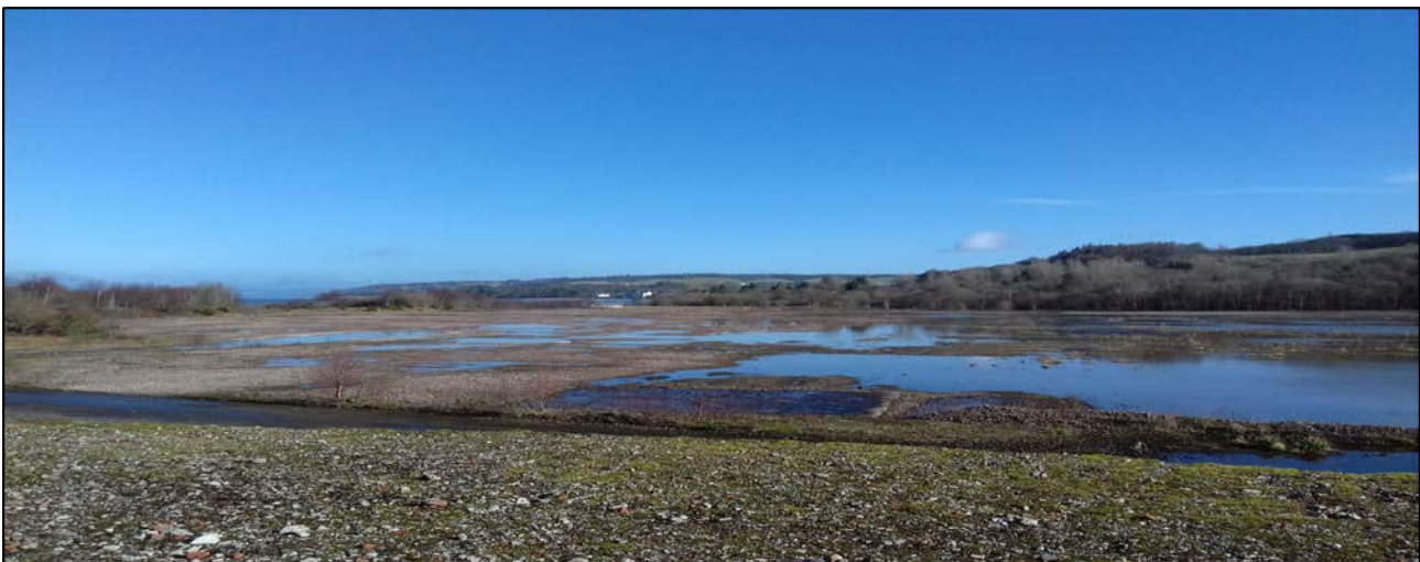
View from elevated position in interior of site looking north
