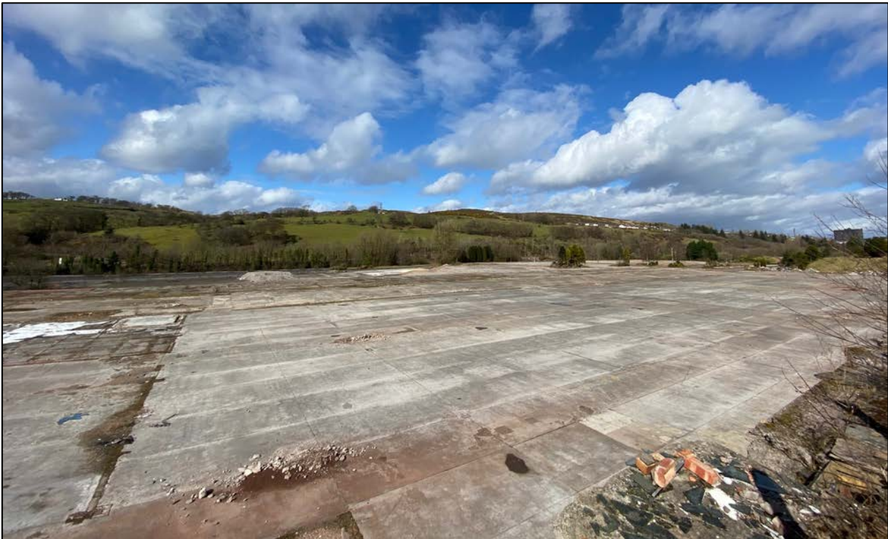
View looking north across the site towards the A78
