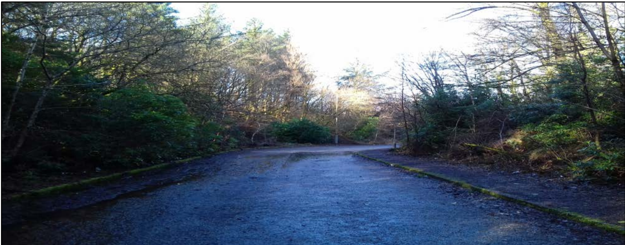
Access road leading down into the site at bend in road before the former power station gatehouse
